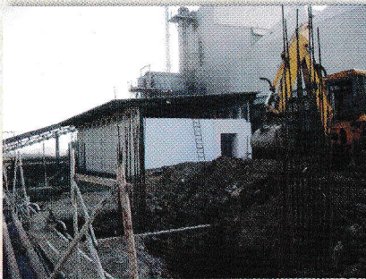
Construction Work In Full Swing
