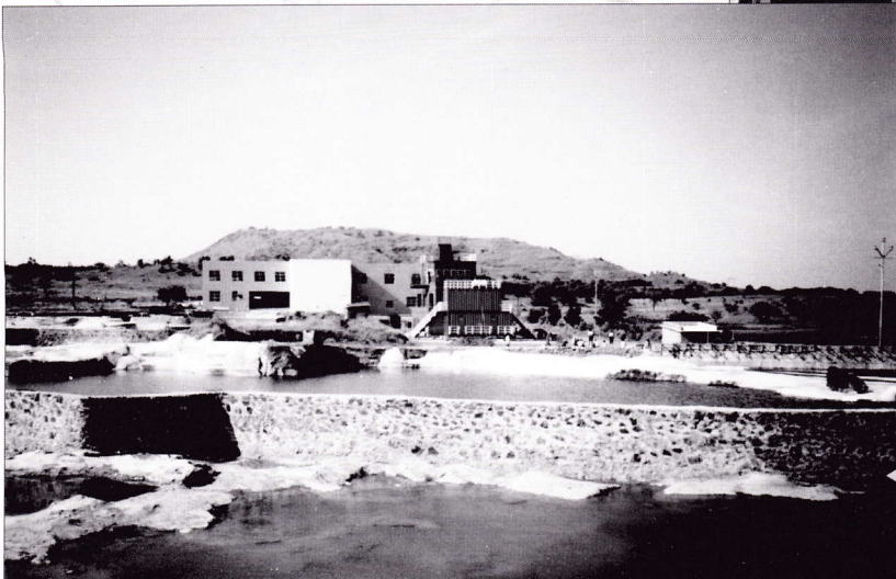
The east block and the fire fighting mockup
