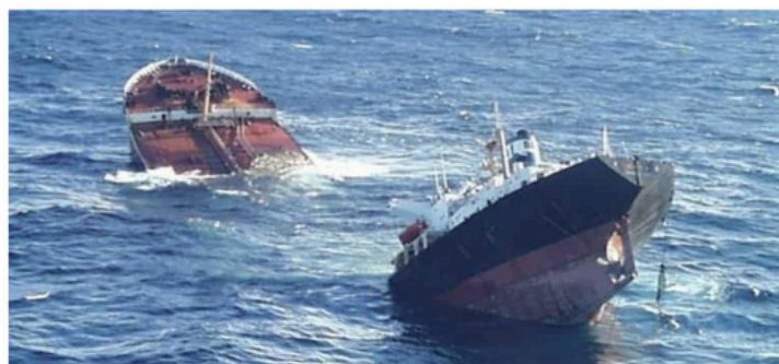
Fig. 1 Structural Failure of the Prestige Tanker
