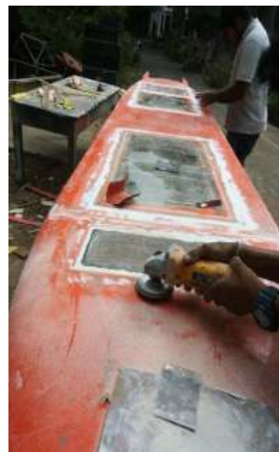
Fig. 12. Smoothening of putti using grinder
