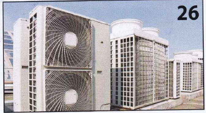
Upgrading Your Current Old Chiller
