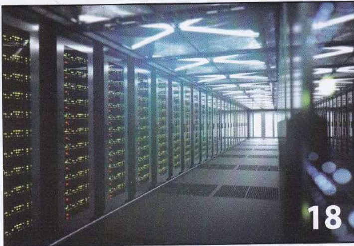
Cover Story: The Future of Data Center Cooling
